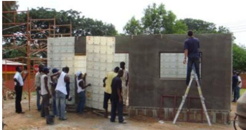
Zero Waste Construction building technology
