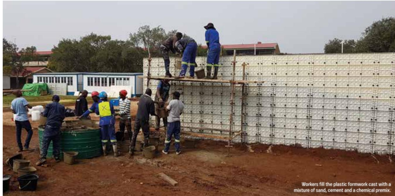
Workers fill the plastic formwork cast with a mixture of sand, cement and a chemical premix.
